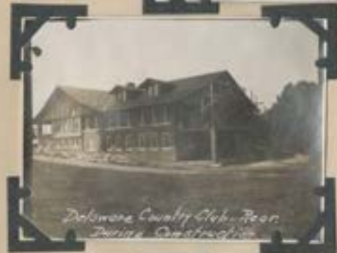
Delaware Country Club, During Construction
