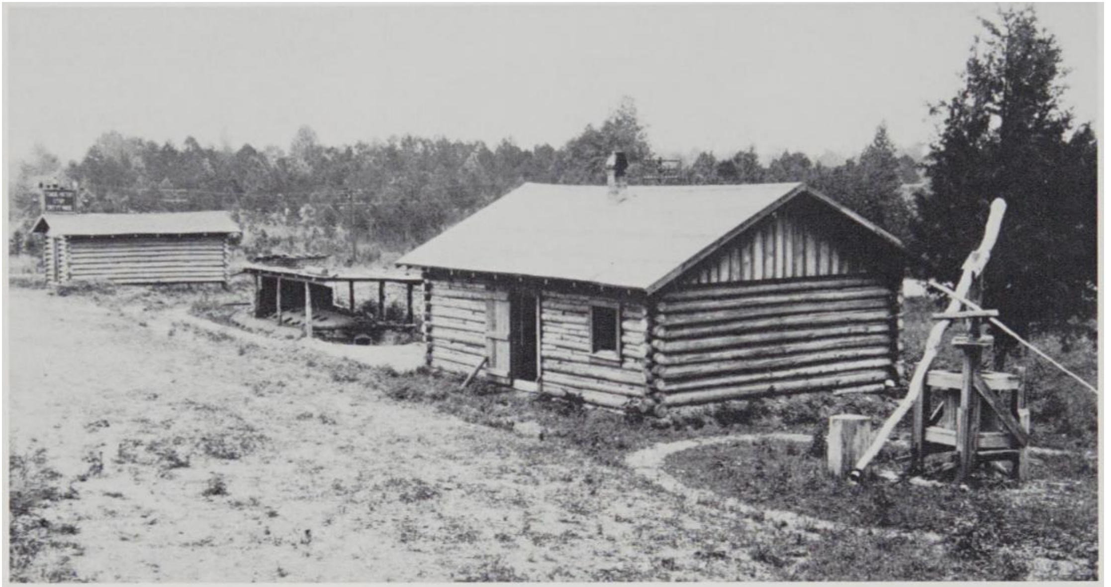
Figure 2-27. The Teague Pottery near Robbins, Moore County [North Carolina], ca. 1930. From left to right are the sales cabin (a feature not seen on the older potteries), the groundhog kiln, the shop, and the mule-powered clay mill. Courtesy of the Teague Family [From Zug, Charles 2000 Turners and Burners: The Folk Potters of North Carolina, pg. 58]
