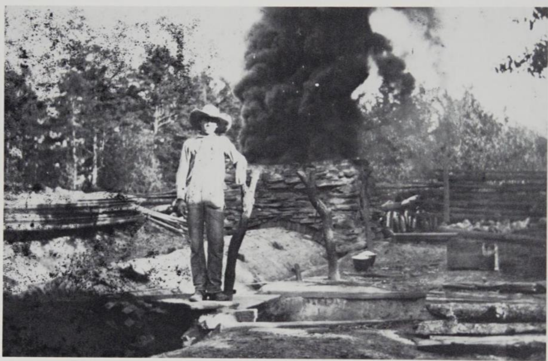
Figure 6-5. The groundhog kiln at the pottery of Baxter N. Welch, Harper's Crossroads, Chatham County [North Carolina], ca. 1900. Courtesy of Mr. and Mrs. Gails Welch [From Zug, Charles 2000 Turners and Burners: The Folk Potters of North Carolina, pg. 172]
