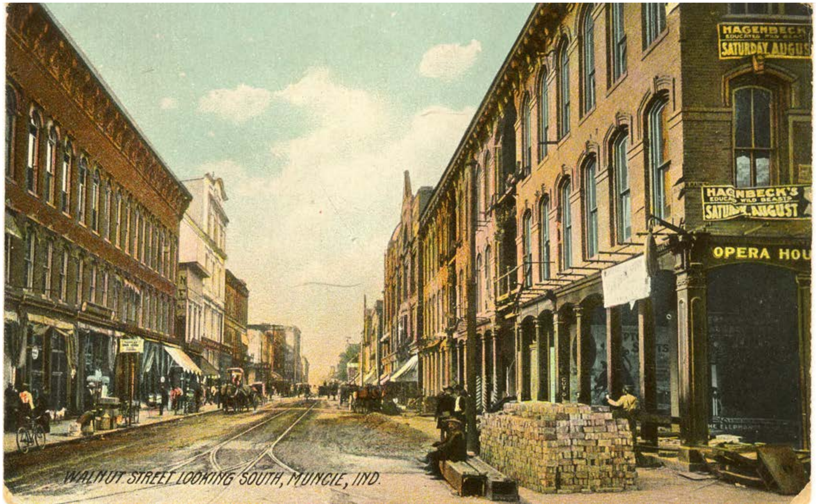
Muncie had a thriving downtown in the late 19 th and early 20 th Centuries, centered on several blocks of south Walnut Street. Here Walnut Street is being paved with brick.
