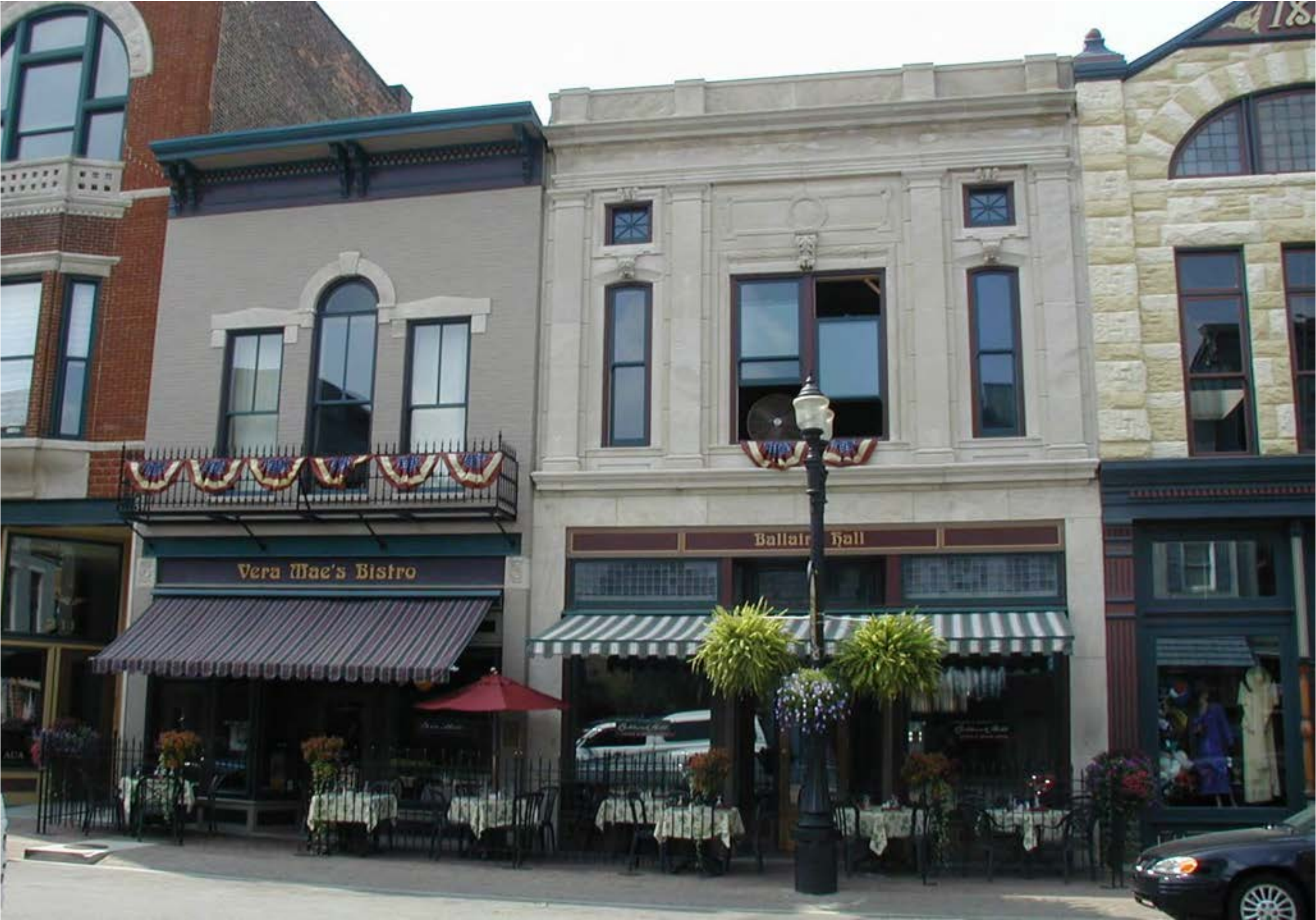
Ballaird Hall completed as an annex to Vera Mae's.
