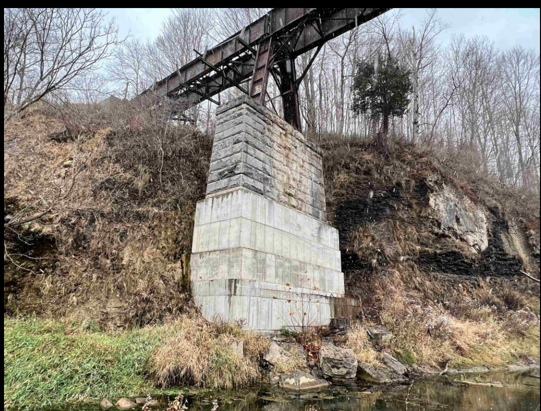
Monon High Bridge Pier Rehabilitation, Carroll County
