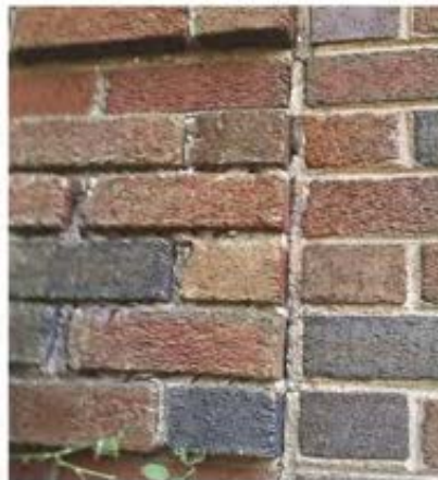
(3) Not Recommended: The white film on the upper corner of this historic brick row house is the result of using a scrub or slurry coating, rather than traditional repointing by hand, which is the recommended method.
