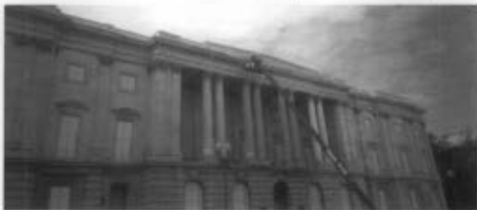
Figure 1. View to southeast exterior corner. Best architectural water repellent is being used to clean the exterior of the U.S. Trust Company Building, a 1914 masonry building constructed in Washington, D.C., in 1914. The building was selected by the architectural conservator as the "perfect" water repellent to clean the masonry. Stone can often have graying deposits such as those on the upper and column capitals, and decorative moldings. Note how these deposits have been removed from the right side of the cornice which has already been cleaned.
