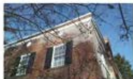
(3) Not Recommended: The white film on the upper corner of this historic brick row house is the result of using a scrub or slurry coating, rather than traditional repointing by hand, which is the recommended method.
