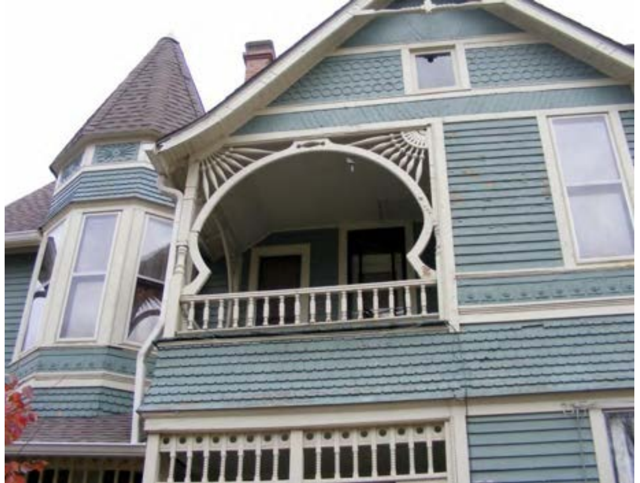
Charles Barr House, Hancock County Good detail photos but...
