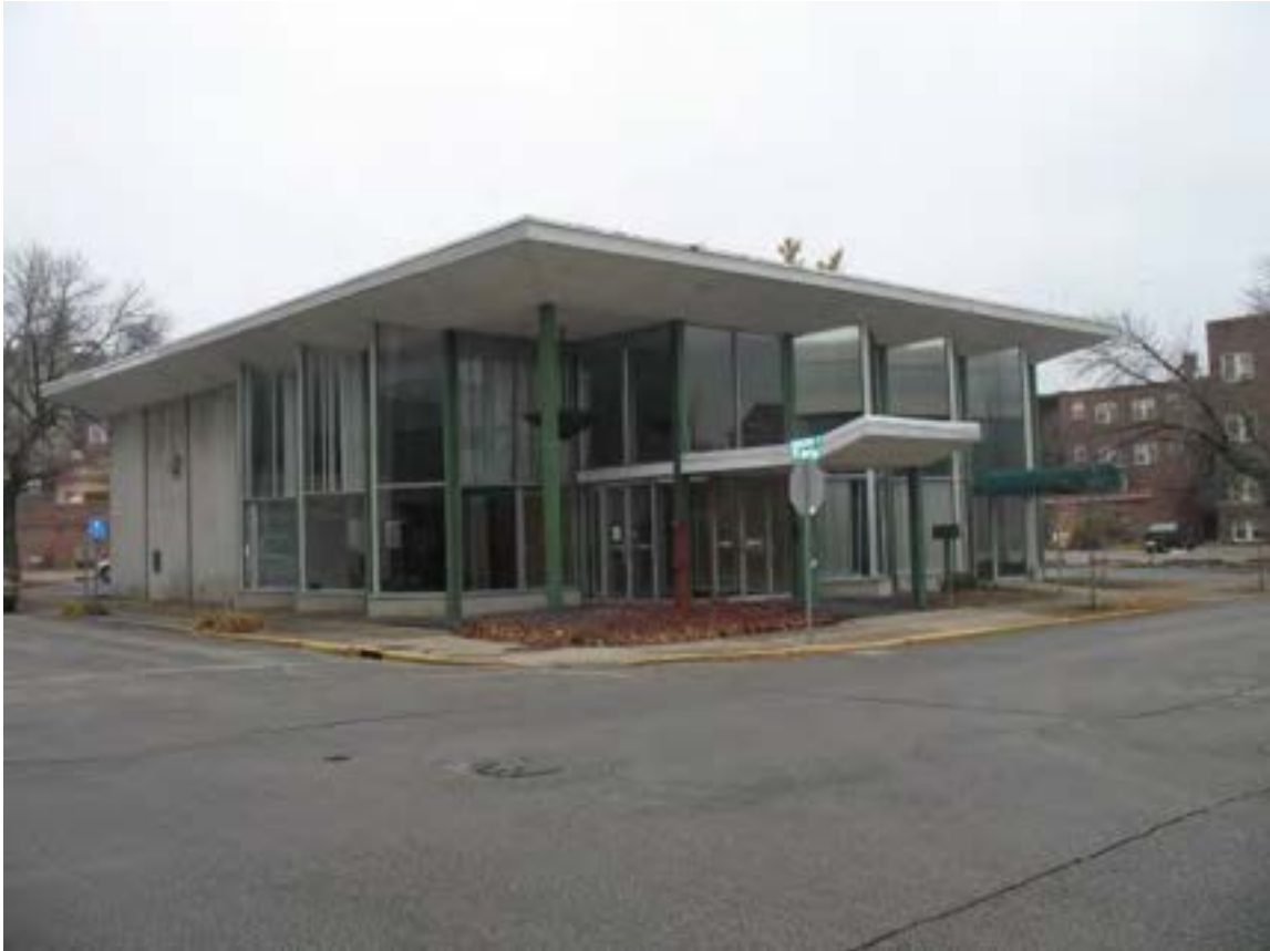
Van Eaton Building Knox County (demolished)
