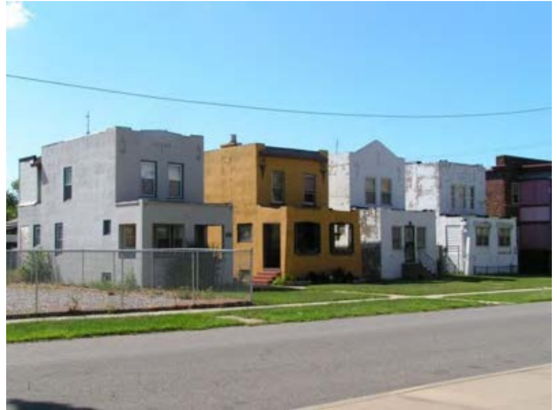
Polk Street Concrete Cottage Historic District, Lake County Criteria A and C/Community Planning and Development, Architecture, and Engineering
