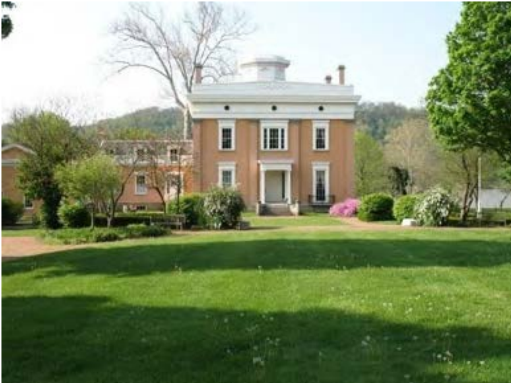
Lanier Mansion, Jefferson County
