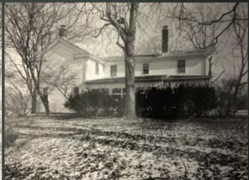
West Elevation Facing US 31
