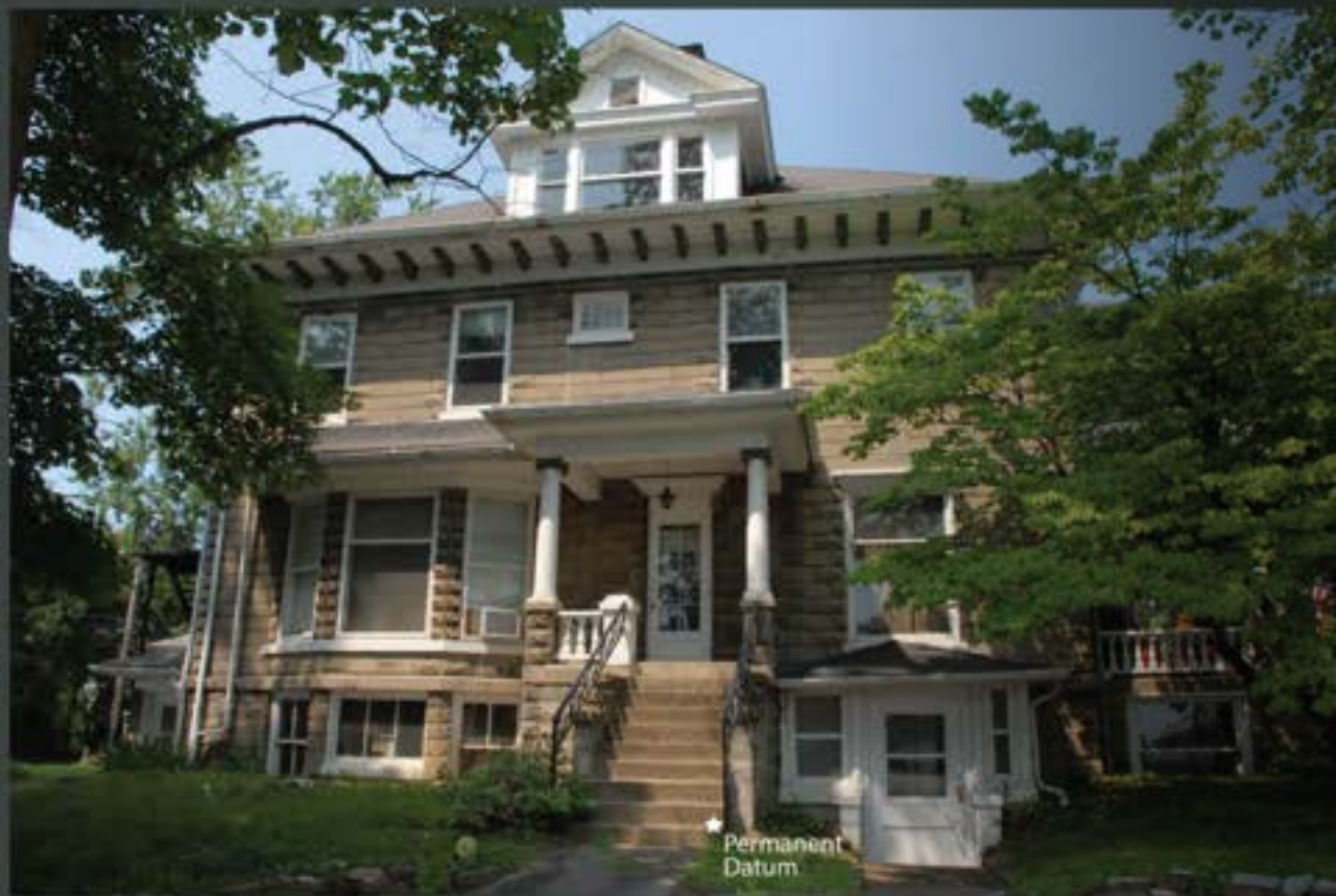
East elevation fronting Market Street
