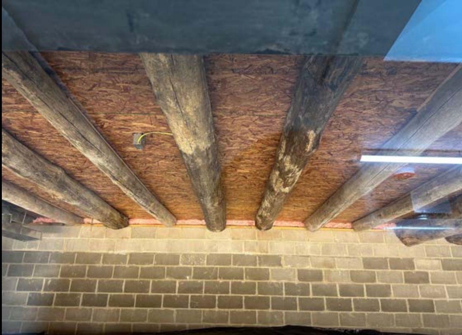
Log joists supporting first floor of house.
