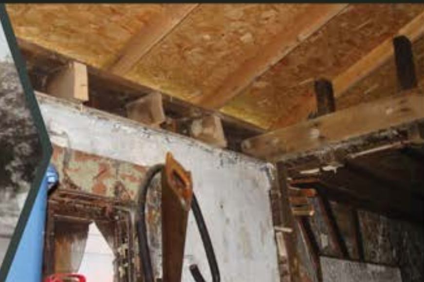
Photograph secured during the field investigation
