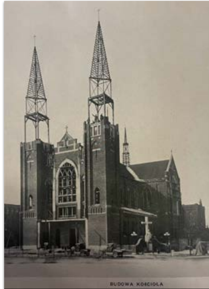
STEEPLES UNDER CONSTRUCTION
