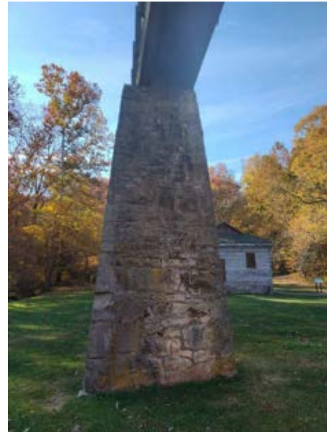
Close up of stone pier with the flume above
