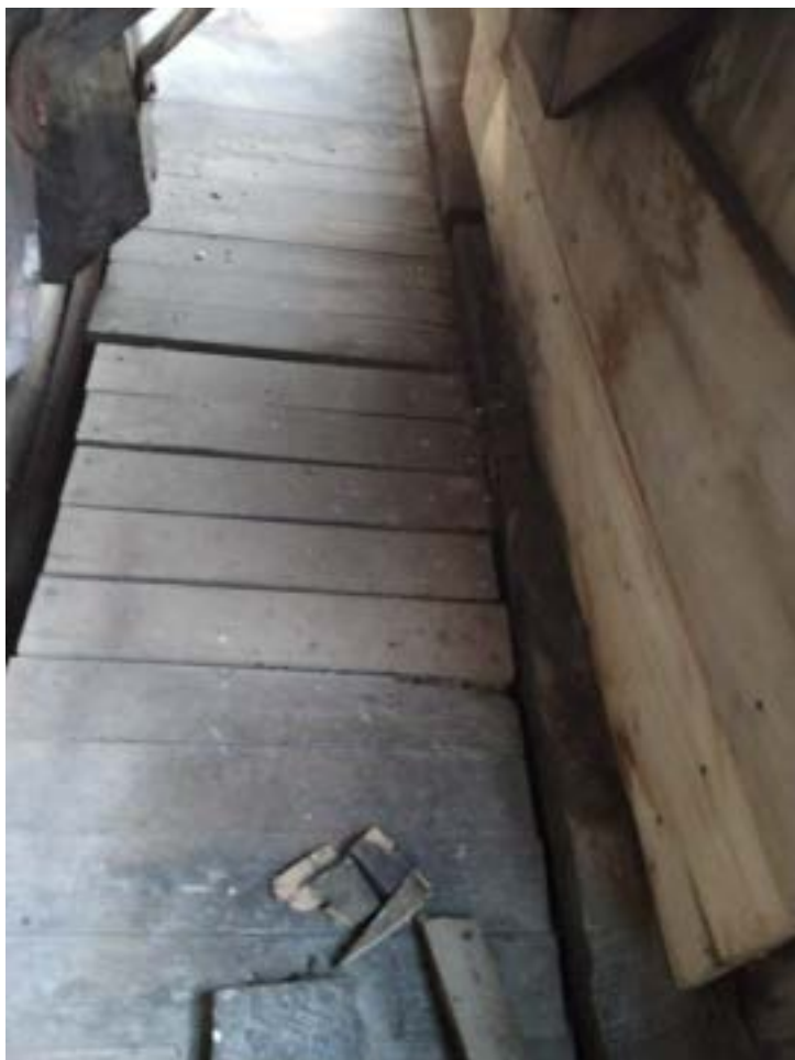
Flooring to be removed to access the damaged sill
