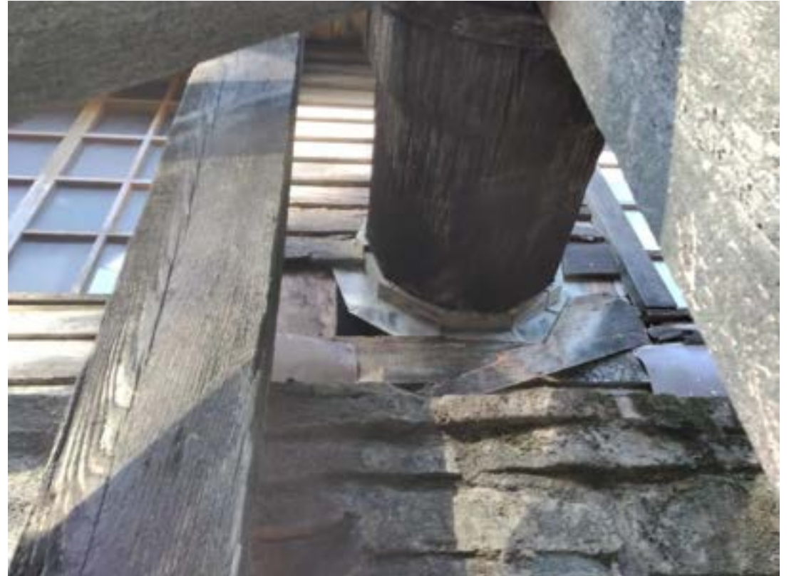
Close up of shaft entrance into mill
