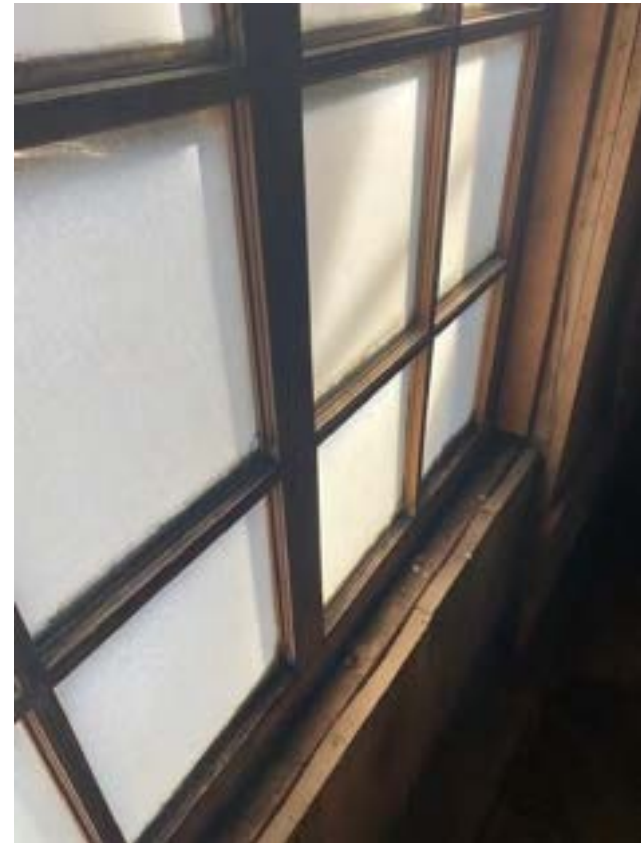
Close up of windows interior view
