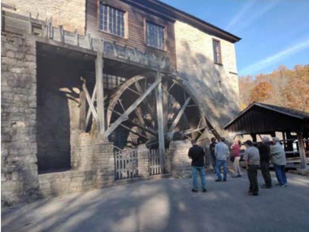
East side of mill, including access and staging area
