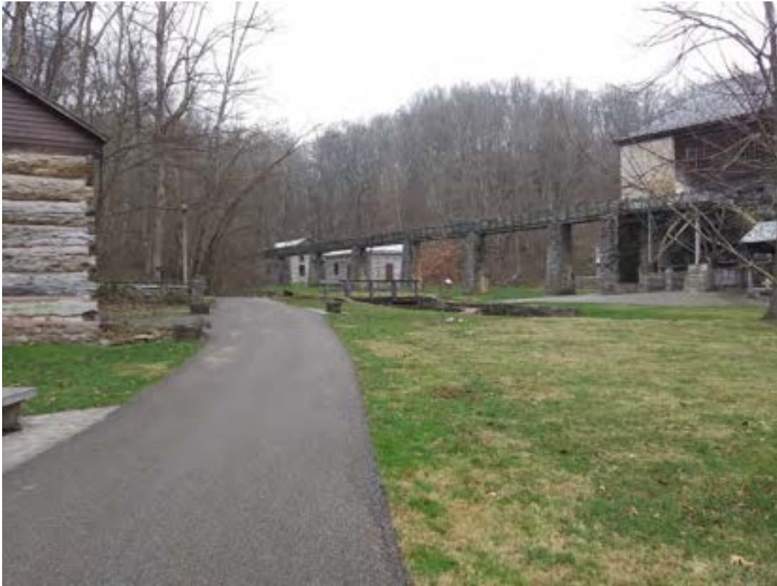
Flume leading from dam to the mill.
