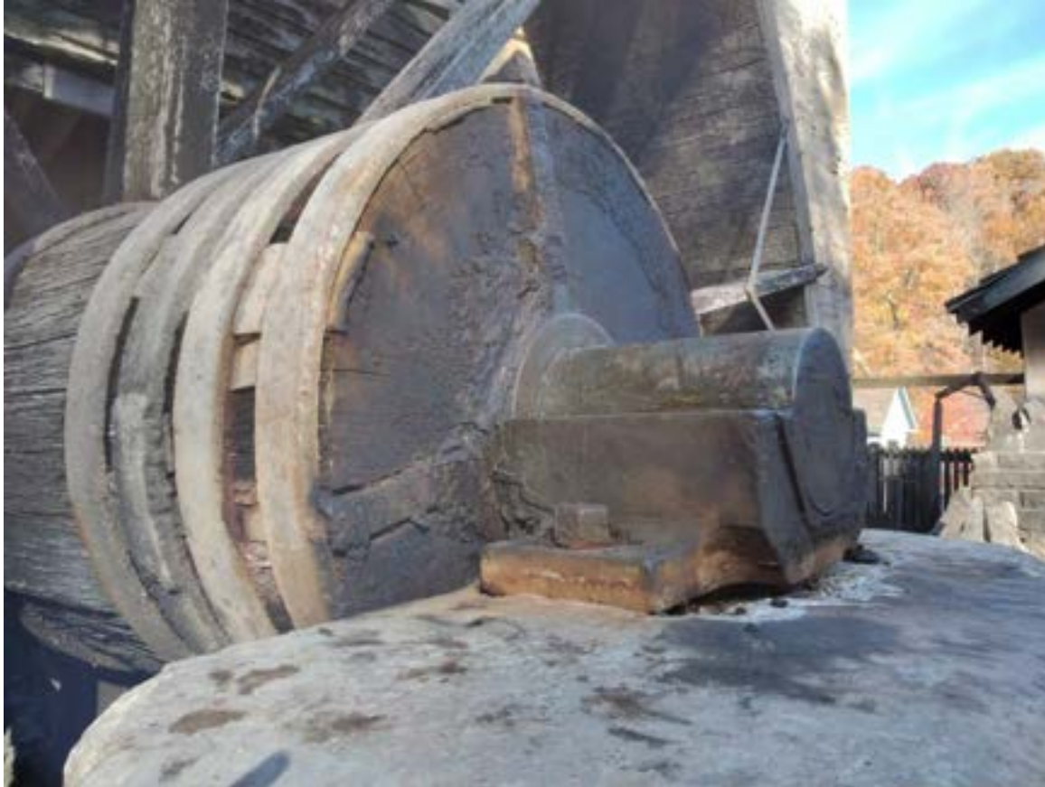
Gudgeon will need to be examined, cleaned, and replaced if needed
