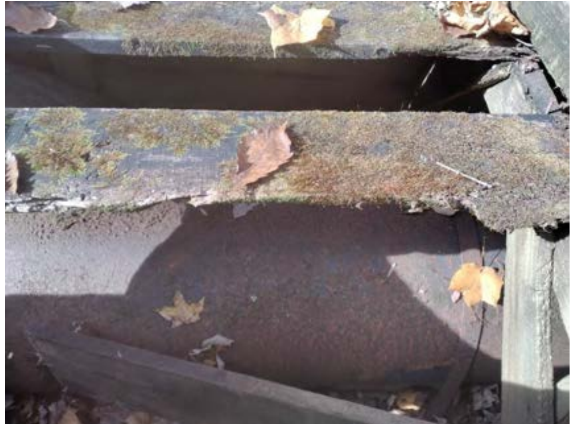
Close up of pipe inside the wooden flume
