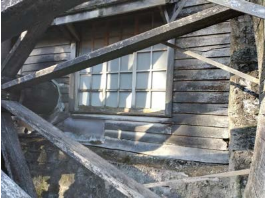
Exterior view of windows and siding
