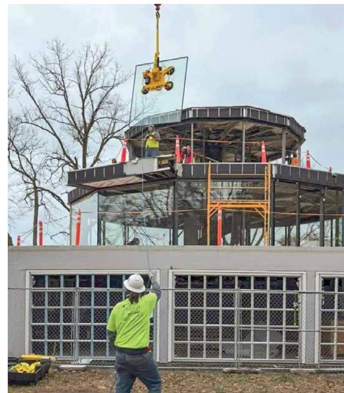
The project reached a milestone in November as workers from Trout Glass guided nearly 1,000-pound panes of glass into place, returning the signature feature of “America’s First Glass House.” The triple-glazed glass fulfills architect George Keck’s original vision of transparent design while also making the structure energy efficient, bringing the “House of Tomorrow” into the modern era.
