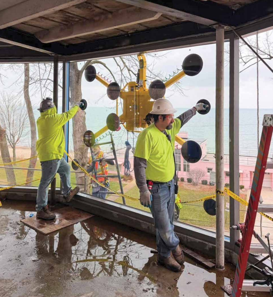
The project reached a milestone in November as workers from Trout Glass guided nearly 1,000-pound panes of glass into place, returning the signature feature of “America’s First Glass House.” The triple-glazed glass fulfills architect George Keck’s original vision of transparent design while also making the structure energy efficient, bringing the “House of Tomorrow” into the modern era.
